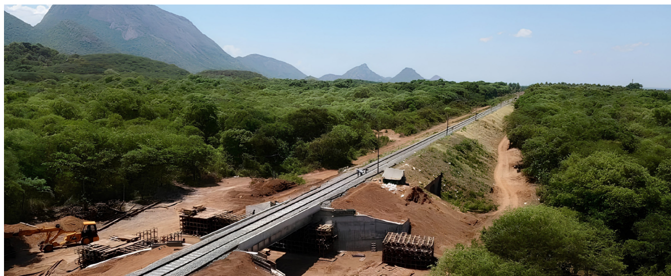
Figure 6. Railway underpass constructed to facilitate safe elephant movement along the Ettimadai-Walayar railway section in Tamil Nadu (Photo credit: Tamil Nadu Forest Department).
