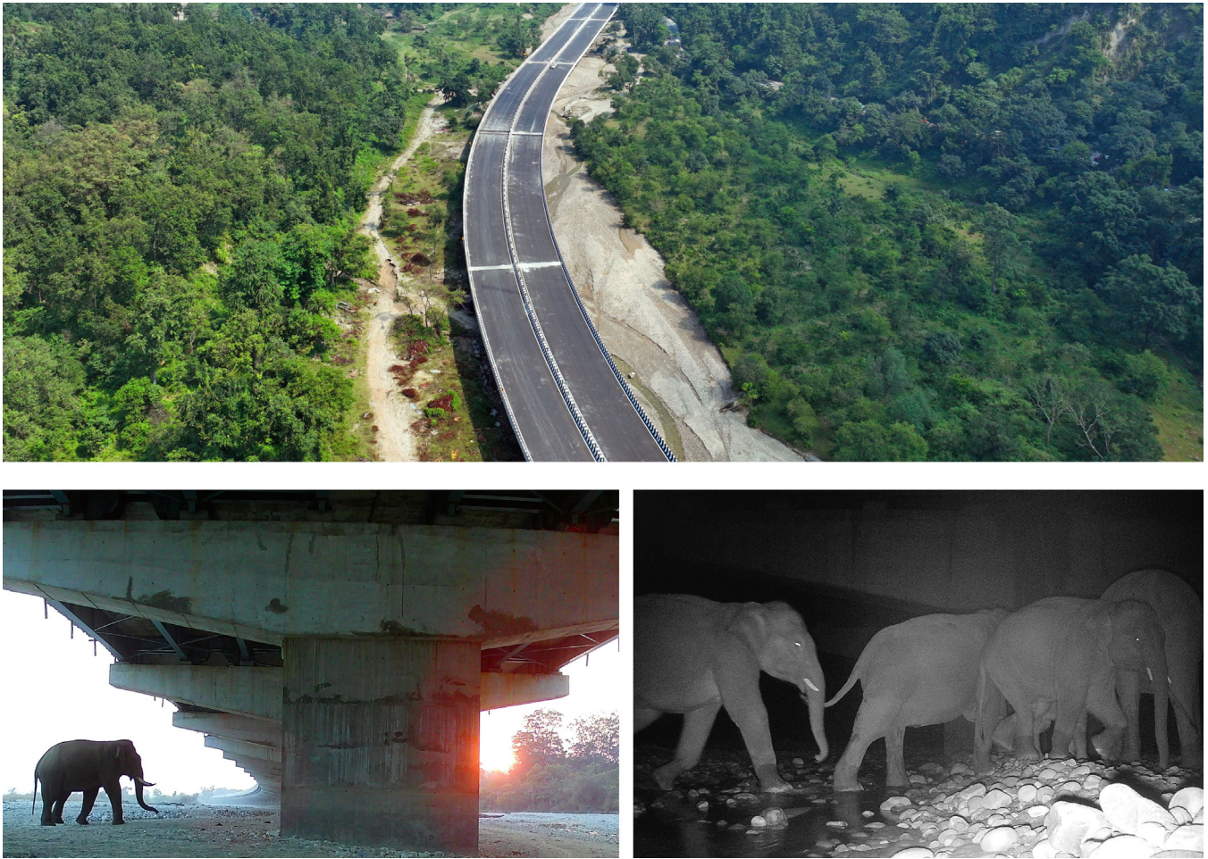
Figure 7. Wildlife underpass on NH-307, Delhi–Dehradun Expressway, one of the world’s largest wildlife viaduct/underpass. The structure is regularly used by elephants and at least 18 other wildlife species, demonstrating its effectiveness in maintaining habitat connectivity and facilitating safe movement for animals.
